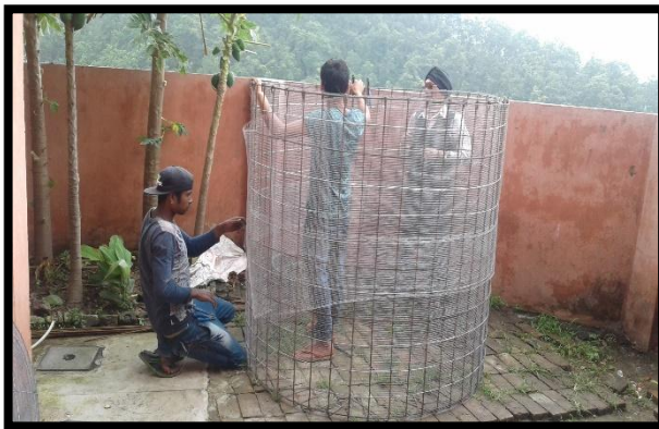
Tank Frame covering with Net
