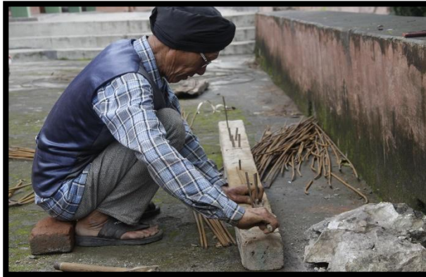
Molding Iron Rod for Tank Frame
