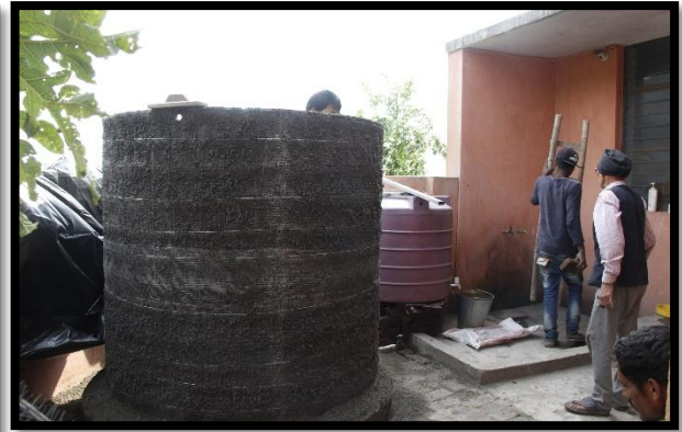
Plastering on Tank frame
