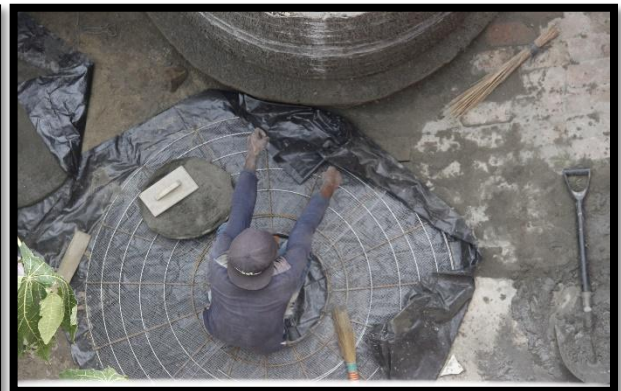
Tank Lid Preparation
