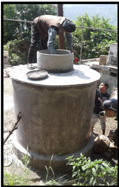
Tank Finishing and Filter fitting
