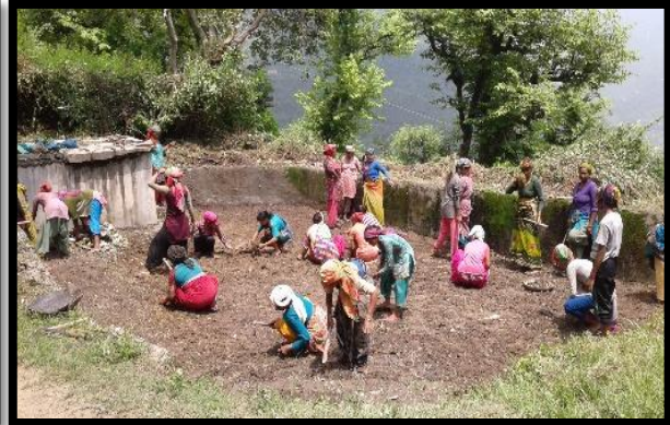
Small Pond 8 Construction at Pipleth
