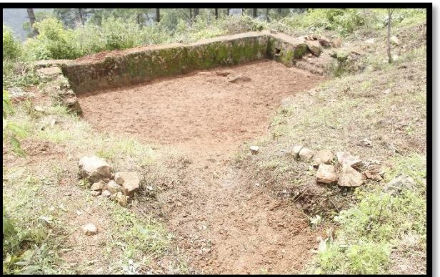
Small Pond 6 Construction at Pipeleth
