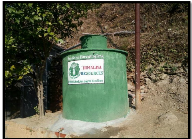
Complete Roof / Rain Water Harvesting Ferro Cement Tank
