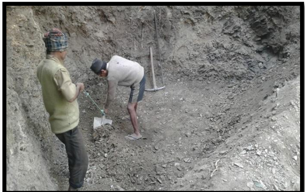
Small Pond 4 Construction at Bhandargau
