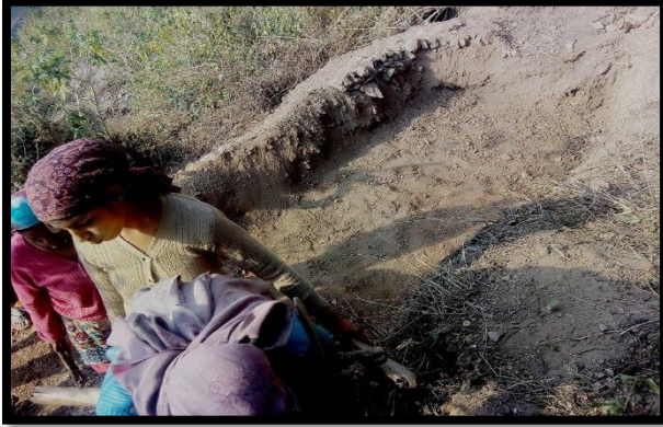
Small Pond 1 Construction at Chidiyali
