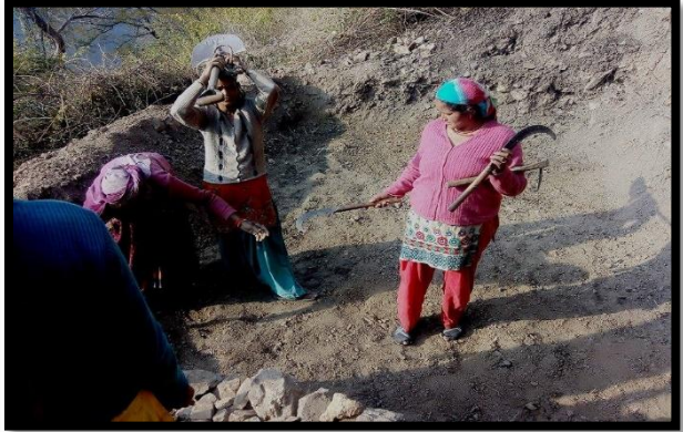
Small Pond 2 Construction at Chidiyali
