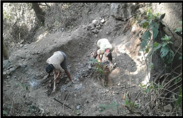
Small Pond 3 Construction at Bhandar Gaun
