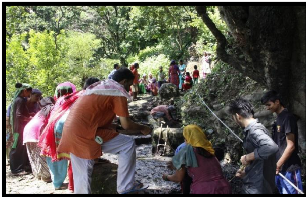
Small Pond 9 Construction at Kathiya
