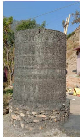
Construction of Roof/Rain Water Ferro Cement Tank
