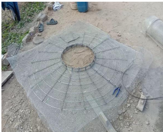
Construction of Roof/Rain Water Ferro Cement Tank
