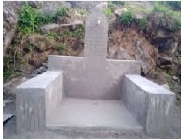
Water tap after the Construction in Sarpang
