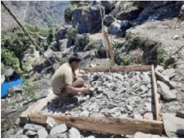
Water tap during construction in Sarpang
