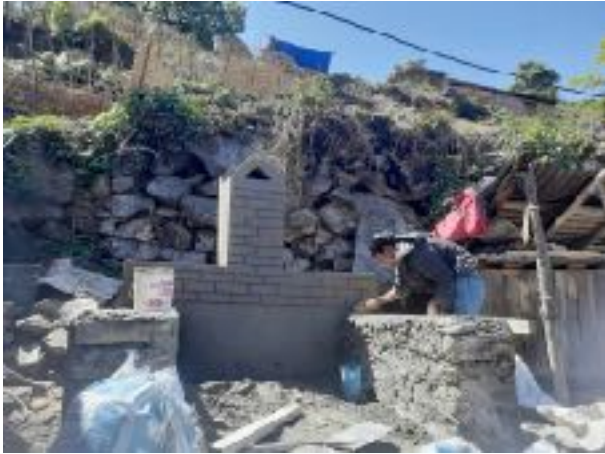
Water tap during construction in Sarpang
