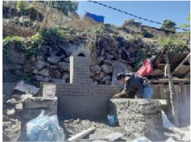
Water tap during construction in Marming
