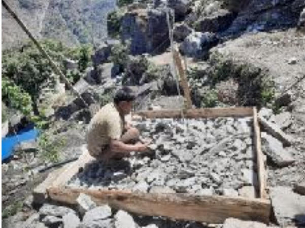
Water tap during construction in Marming
