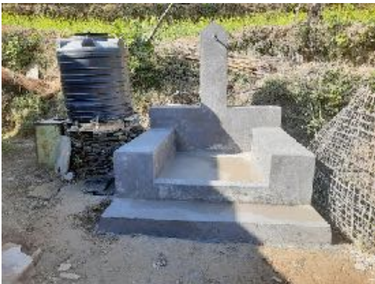
Water tap after the construction
