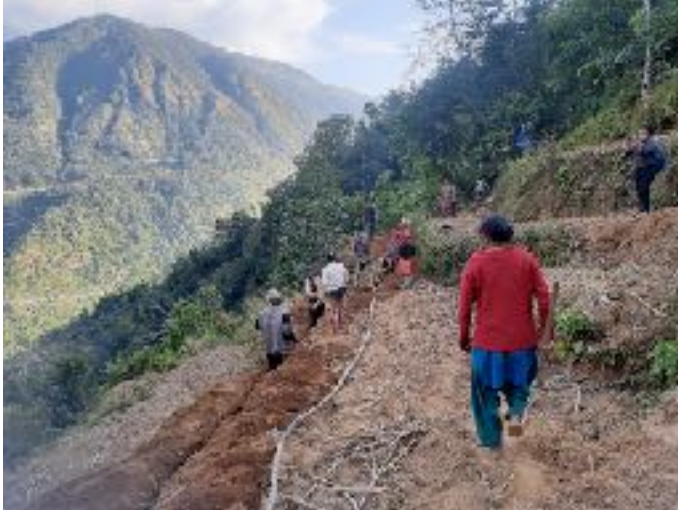
Villagers digging the pathway for the Pipeline in Ghumthang
